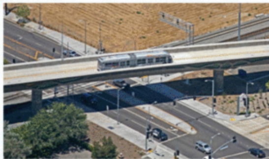
Los Angeles County Metropolitan Transportation Authority, Orange Line Extension Design-Build Los Angeles County, California
