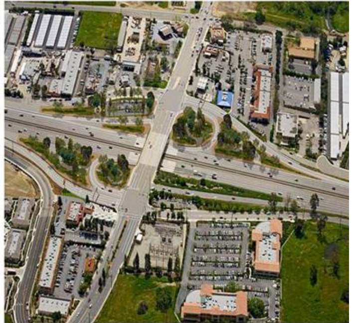
Kanan Road Interchange—Agoura Hills, CA
